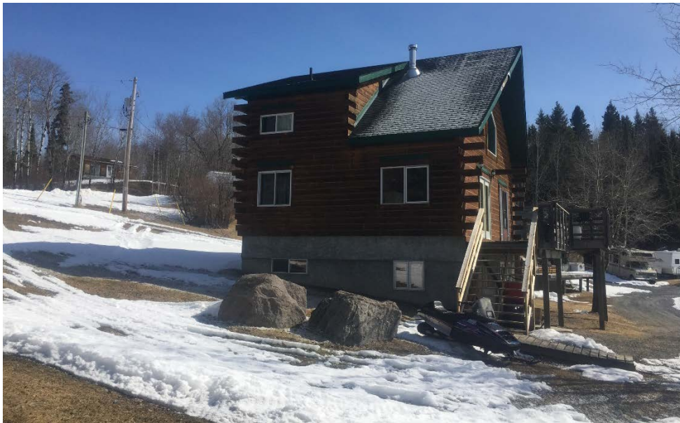
Photo 5 – West most cabin
